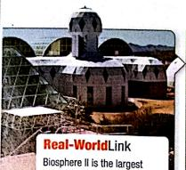
Biosphere II is the largest totally enclosed ecosystem ever built, covering 3.14 acres in Oracle, Arizona. The controlled-environment facility is 91 feet at its highest point, and it has 6500 windows that enclose a volume of 7.2 million cubic feet.
